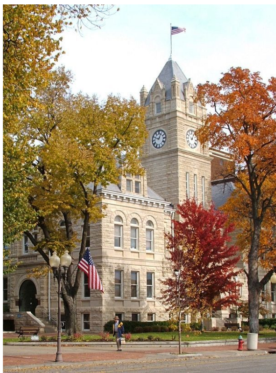
Courthouse built of limestone in Manhattan, Kansas
