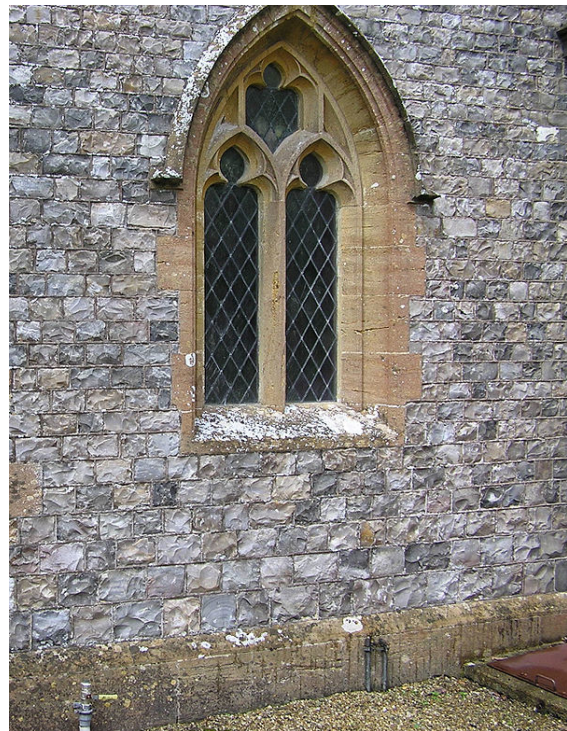
A flint church - the Parish Church of Saint Thomas, in Cricket Saint Thomas, Somerset, England. The height of the very neatly knapped flints varies between 3 and 5 inches (7.6 and 12.7 cm).
